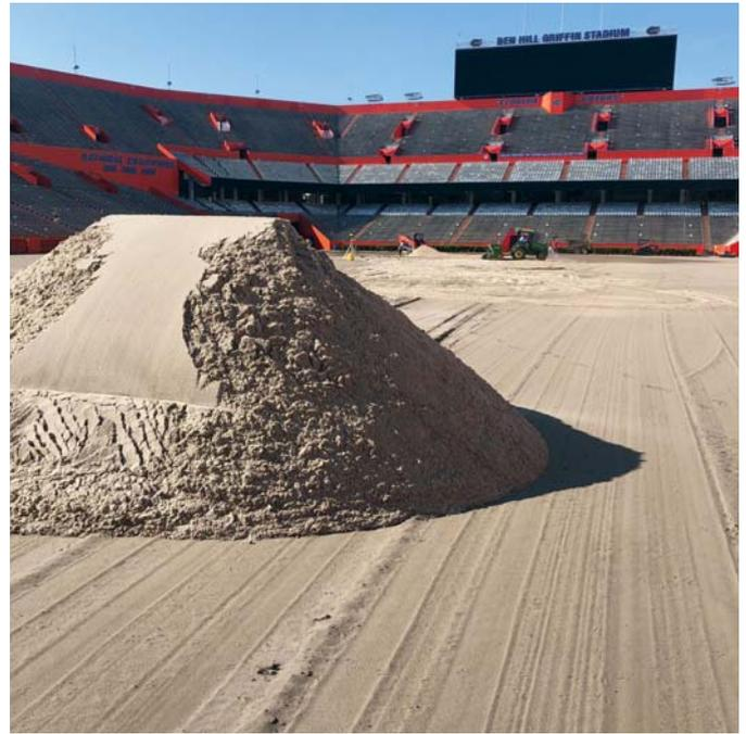
After the existing rootzone material was removed, the new rootzone material consisting of 90 percent USGA sand and 10 percent COMAND was delivered.
